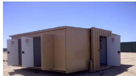
SuperCLU folding structure with easy set up and tear down; transported as an International Standards Organization container
